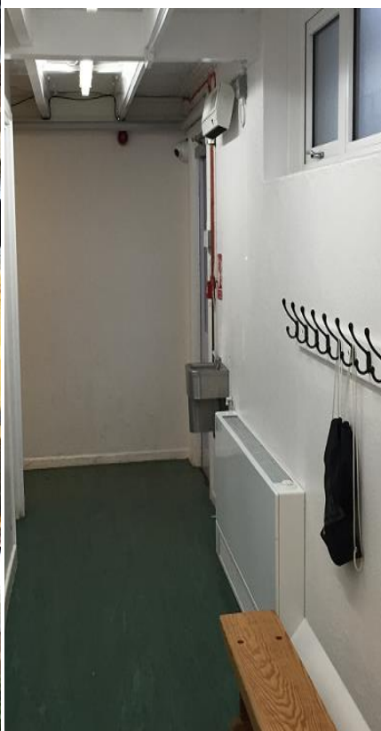
Changing area – this has been disconnected as children change here
